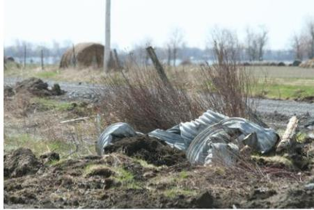
*Culverts were crushed, ditches were filled (Brian Little)*
